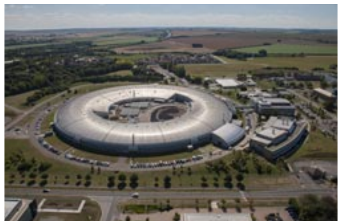
Diamond Light Source Aerial View - Copyright of Diamond Light Source Ltd
